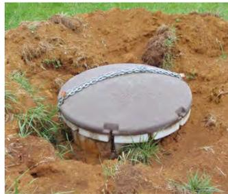
Vault lids were secured with chains and locks before being covered with dirt, like this one at station V51A in Loudon, Tennessee.
