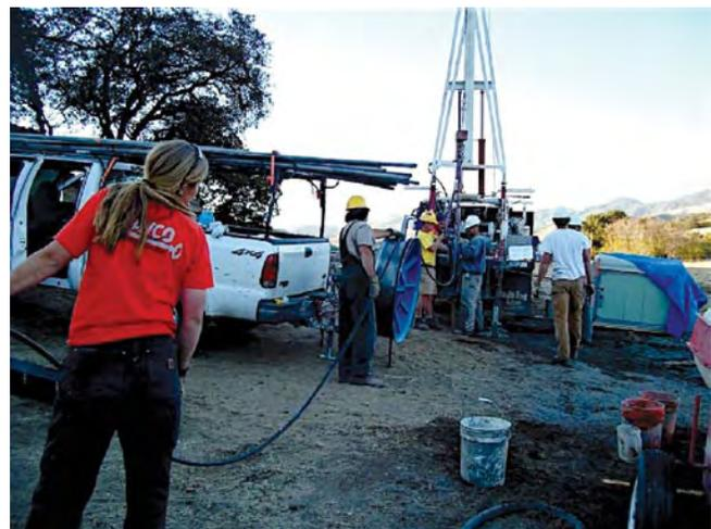
Figure 1.7. A PBO borehole strainmeter/seismometer installation along the San Andreas Fault near Parkfield, California. Engineer in the foreground is spooling out strainmeter cable as the instrument is being lowered into the borehole using the derrick lift in the background.
