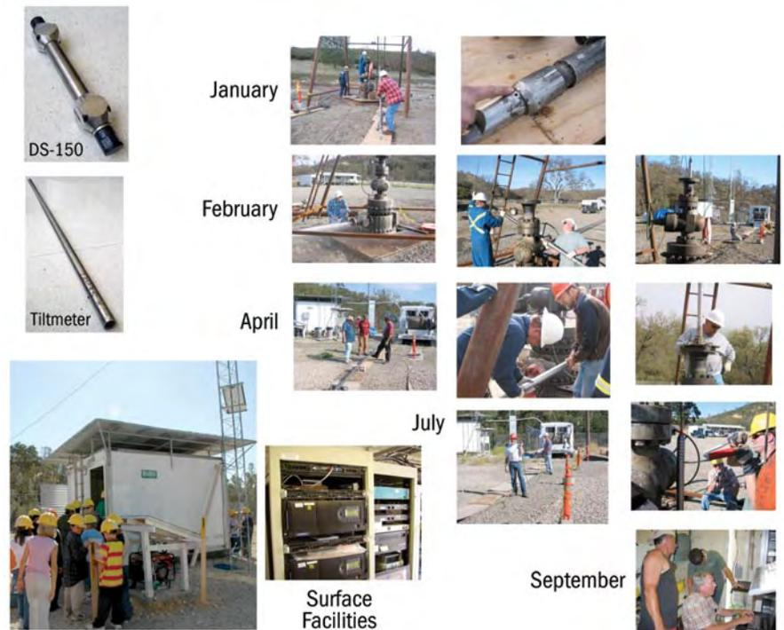
Figure 3.3. A collage of photos related to testing components of the downhole instrumentation systems and the surface facilities instrumentation facilities. A sixth grade class is shown touring the surface instrumentation building. The photo of the instrumentation rack shows the earthworm computers and LT03 tape drives referred to in Volume I. The Geores recording system for the downhole seismometers is visible in the second rack.
