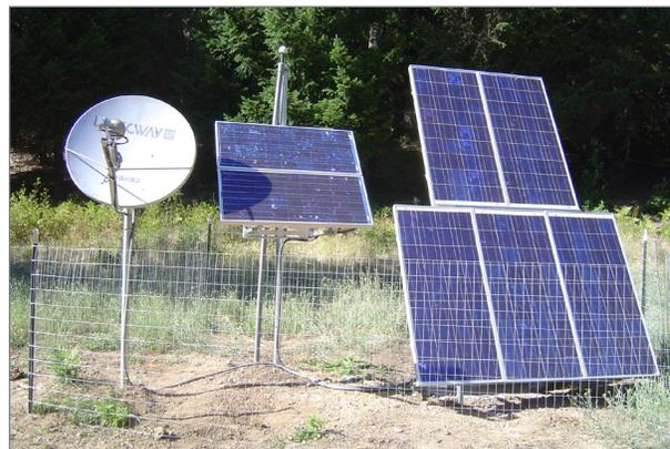
Figure 2-12. TA.N02C operated DC (solar) VSAT with a large bank of solar panels to provide additional power to the communications system
