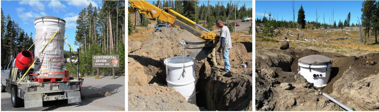
Figure 2-5. Reconstruction of TA.H17A (9/19/11), Yellowstone National Park. The original vault was replaced with a second generation vault to mitigate leaks and achieve better performance.
