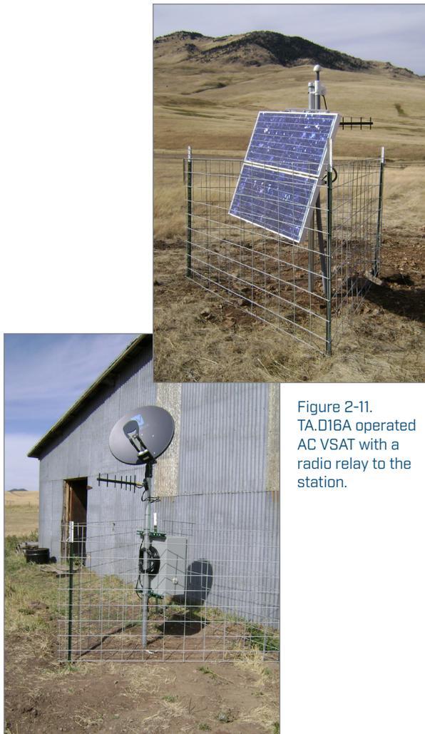
Figure 2-11. TA.D16A operated AC VSAT with a radio relay to the station.
