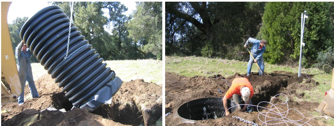
Figure 2-4. Construction of TA.BNLO (3/7/05) using a first generation vault.
