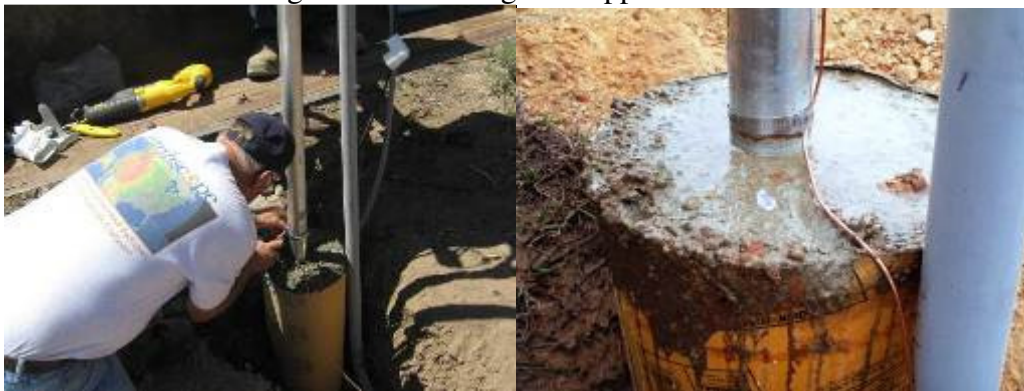
27. Attach ground wire to mast with hose clamp
