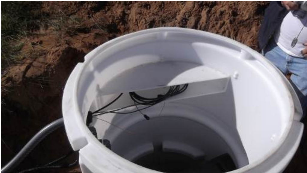
16. Coil comm, GPS, power, and ground cables inside vault
