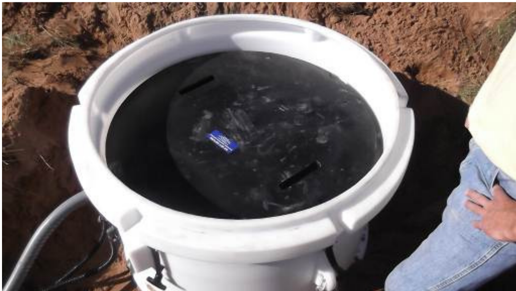
17. Install upper foam in vault.
