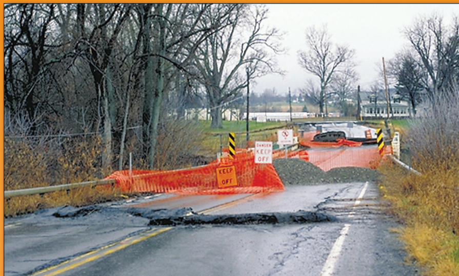
Damage caused by the Retsof Salt Mine Collapse.
